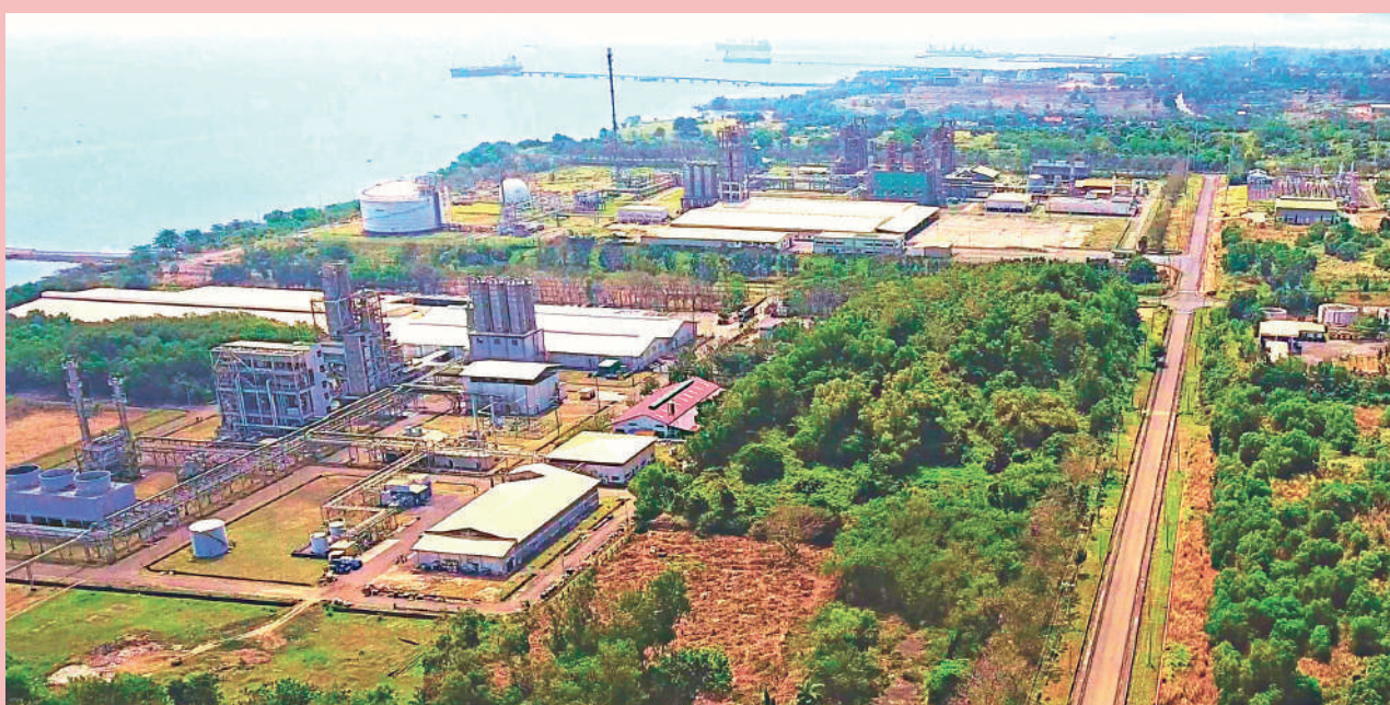
The PNOC Industrial Park
